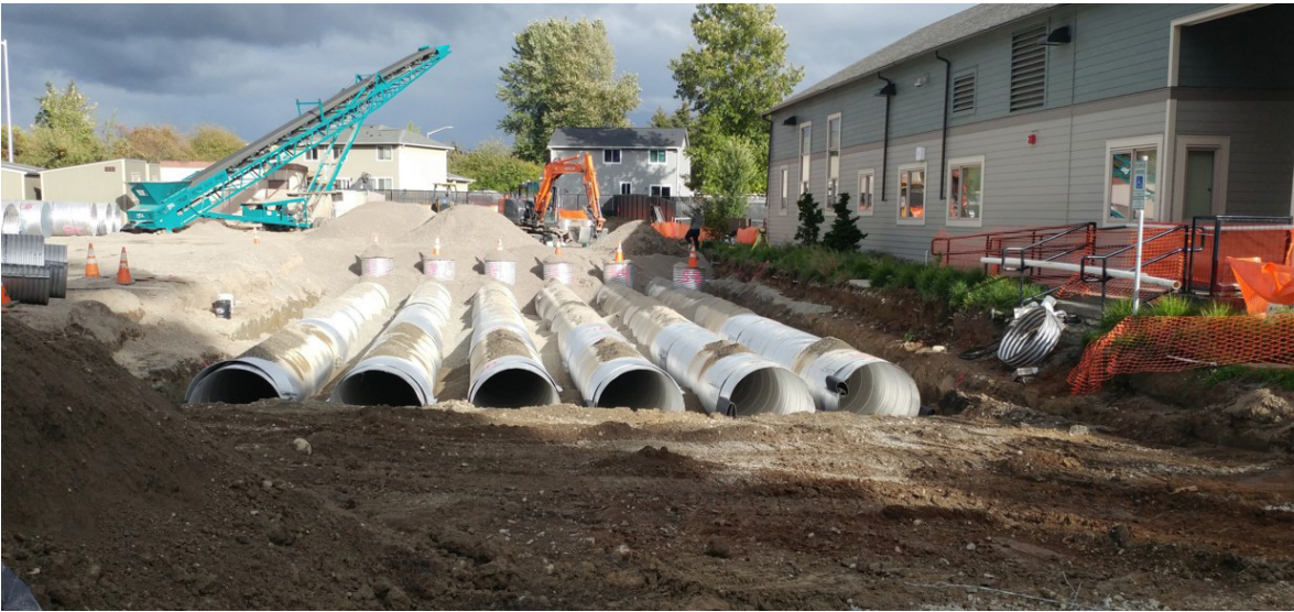
The Dr. Frank Hewins ELC parking lot now has 350,000 gallons of stormwater storage beneath the pavement
